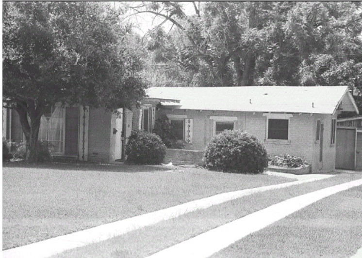
Original survey photo (ca. 1990)
