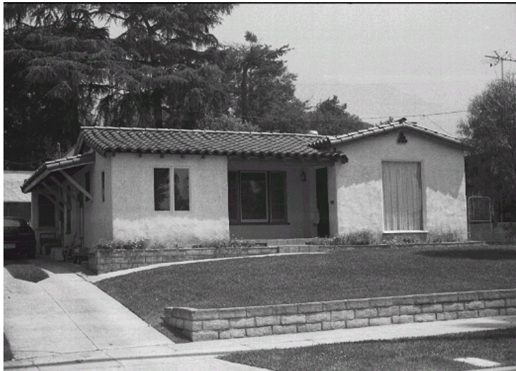
Original survey photo (ca. 1990)
