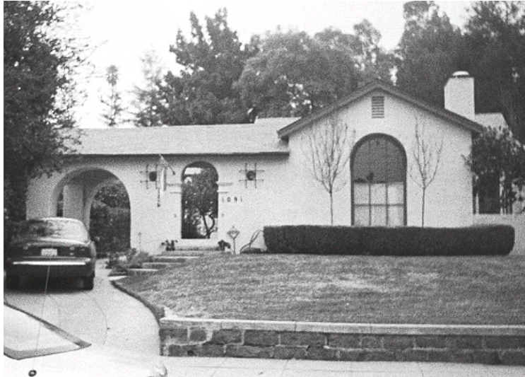
Original survey photo (ca. 1990)
