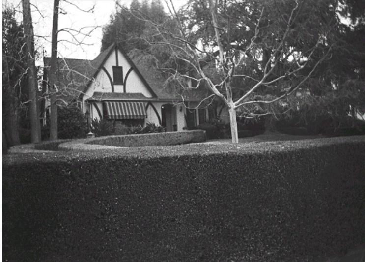
Original survey photo (ca. 1990)
