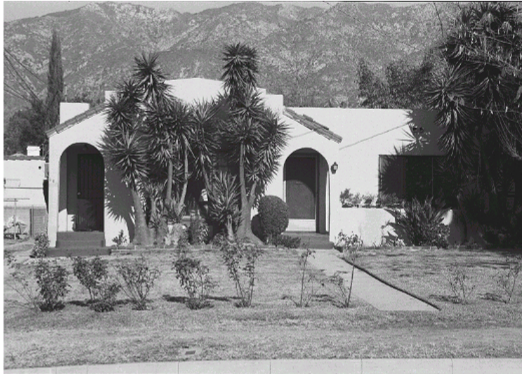
Original survey photo (ca. 1990)
