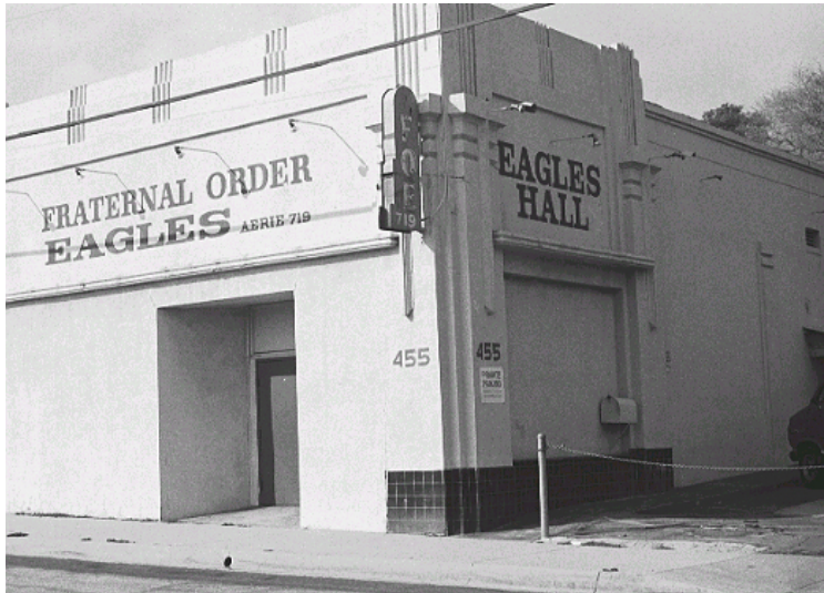
Original survey photo (ca. 1990)
