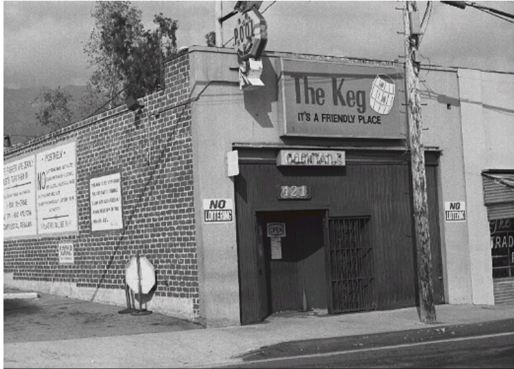
Original survey photo (ca. 1990)
