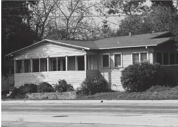
Original survey photo (ca. 1990)
