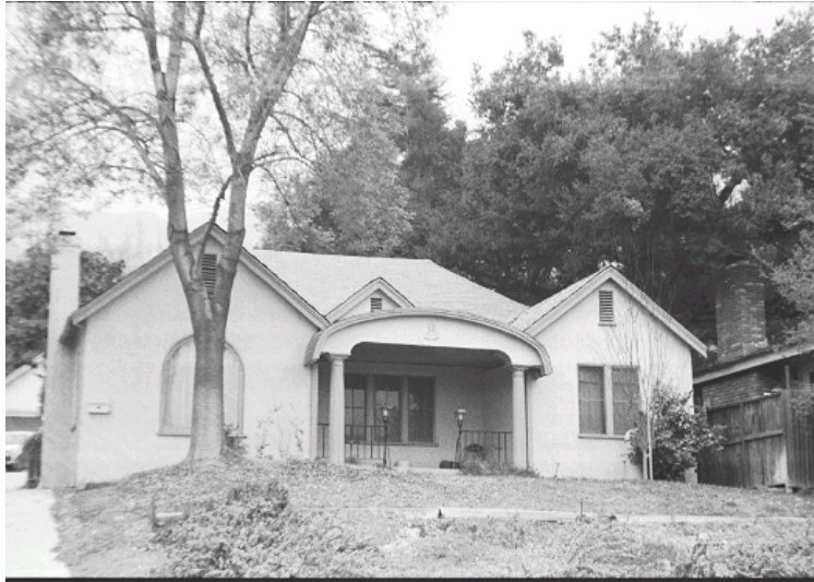
Original survey photo (ca. 1990)
