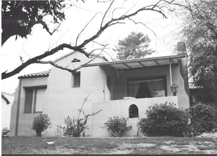
Original survey photo (ca. 1990)
