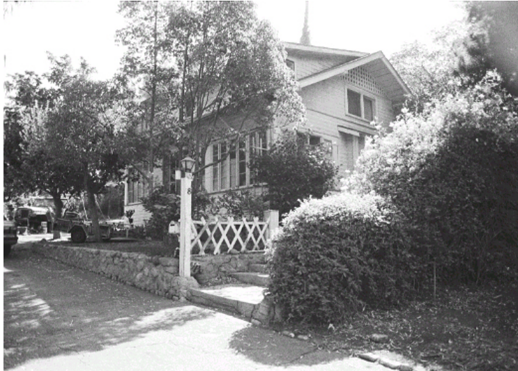
Original survey photo (ca. 1990)
