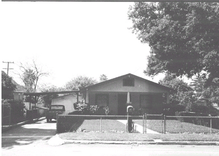
Original survey photo (ca. 1990)
