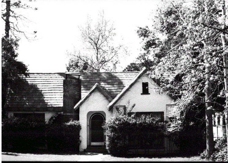
Original survey photo (ca. 1990)
