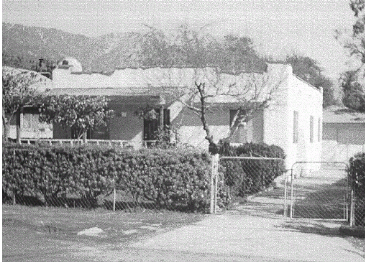
Original survey photo (ca. 1990)
