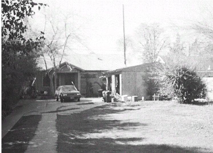
Original survey photo (ca. 1990)
