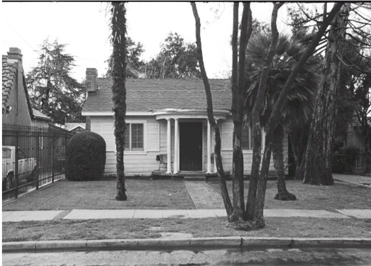
Original survey photo (ca. 1990)
