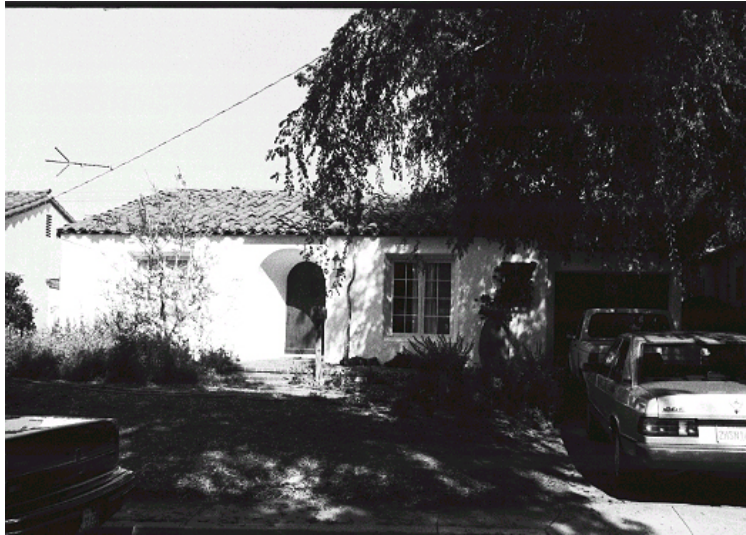
Original survey photo (ca. 1990)
