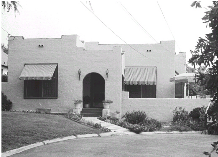
Original survey photo (ca. 1990)
