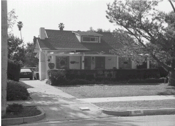
Original survey photo (ca. 1990)
