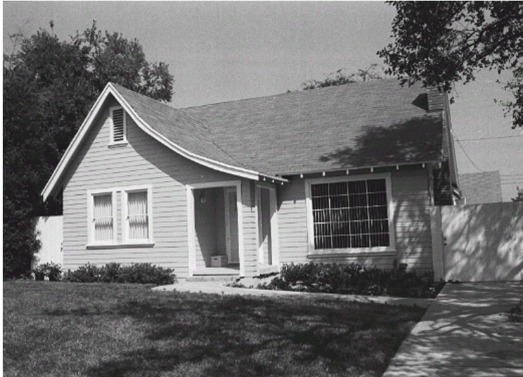
Original survey photo (ca. 1990)
