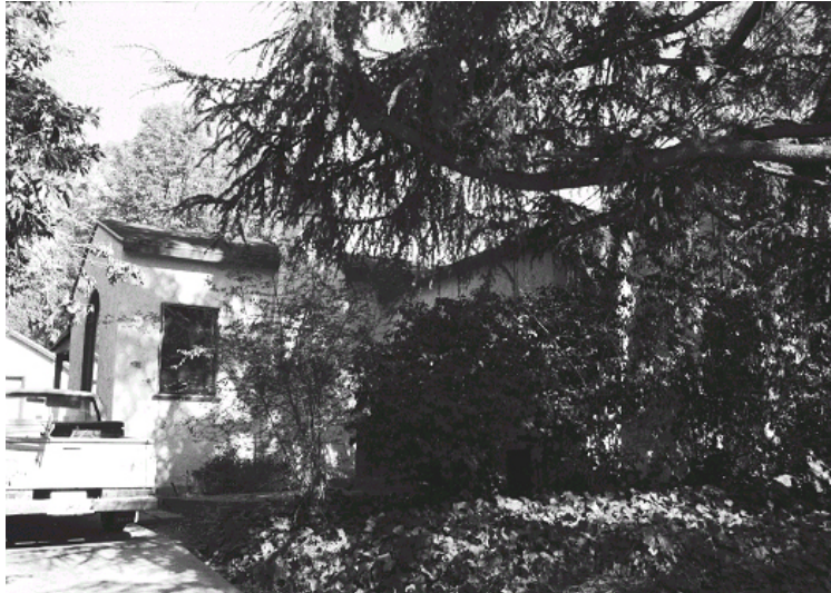
Original survey photo (ca. 1990)
