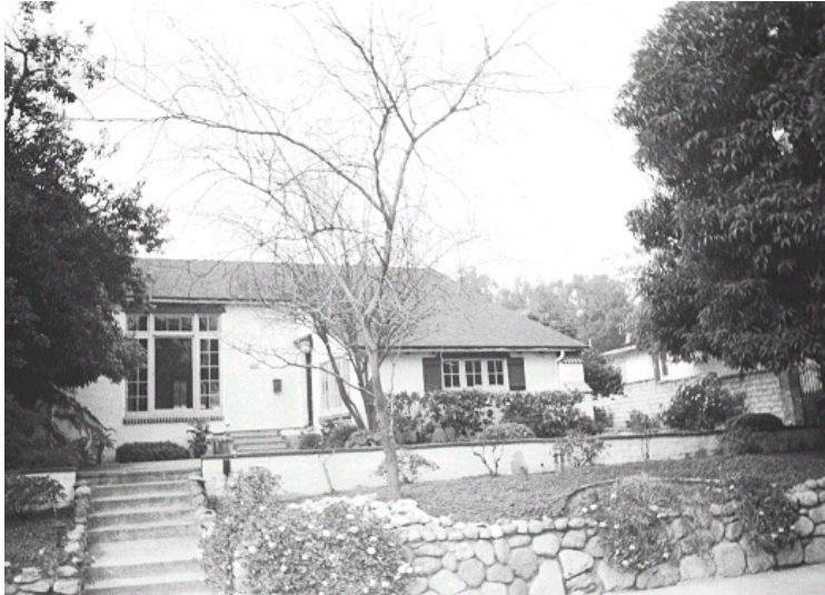
Original survey photo (ca. 1990)
