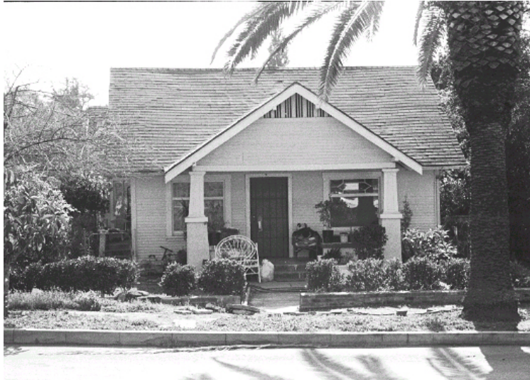
Original survey photo (ca. 1990)
