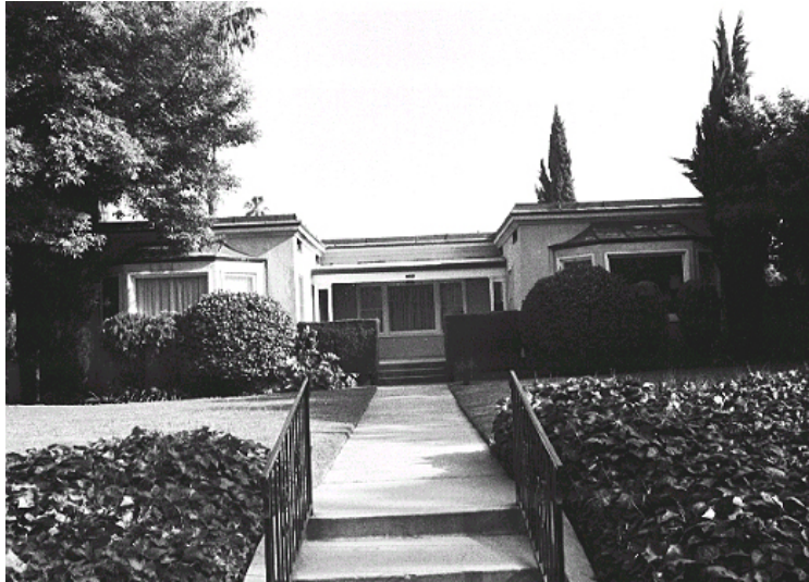
Original survey photo (ca. 1990)
