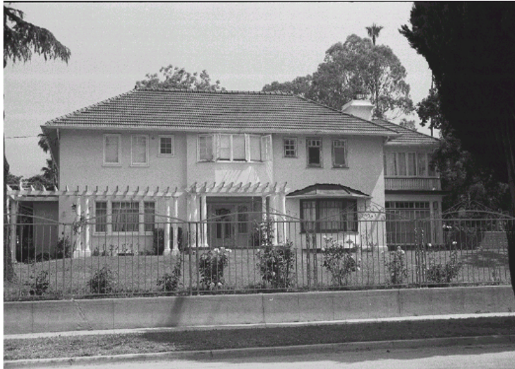
Original survey photo (ca. 1990)
