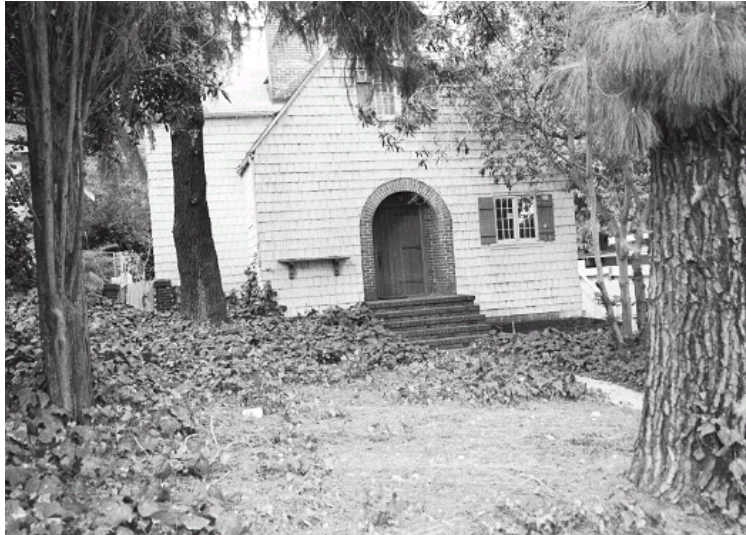
Original survey photo (ca. 1990)
