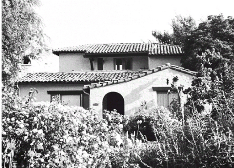
Original survey photo (ca. 1990)
