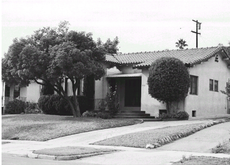
Original survey photo (ca. 1990)
