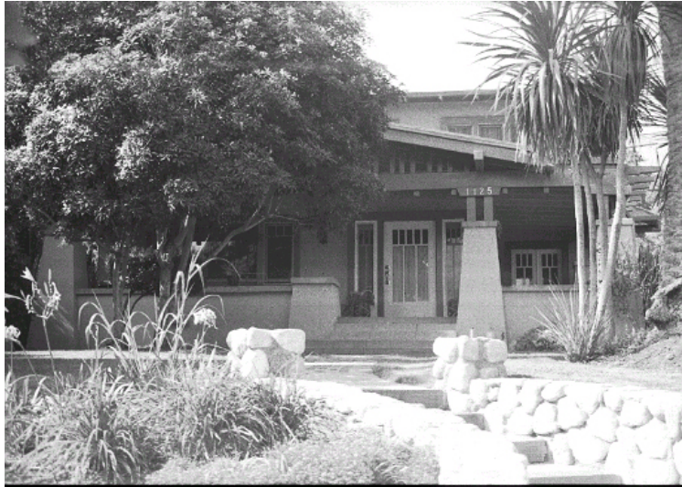
Original survey photo (ca. 1990)
