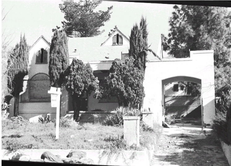
Original survey photo (ca. 1990)
