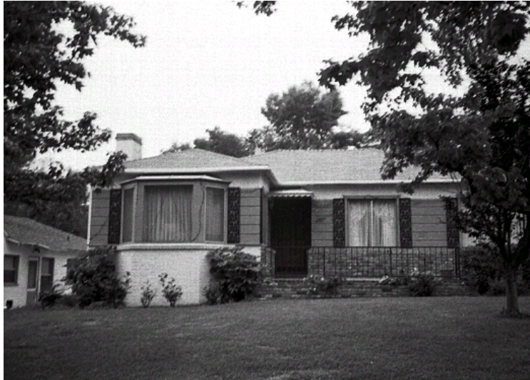
Original survey photo (ca. 1990)
