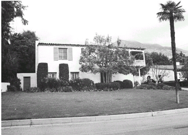
Original survey photo (ca. 1990)
