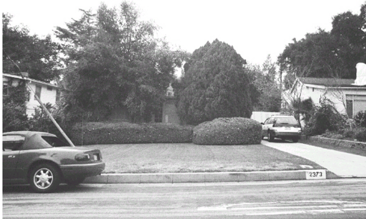
Original survey photo (ca. 1990)
