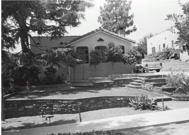
Original survey photo (ca. 1990)
