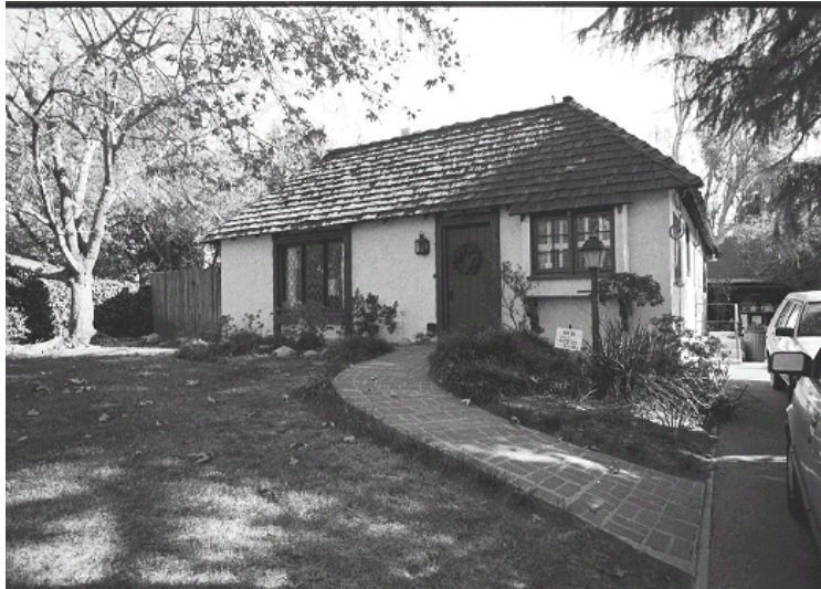
Original survey photo (ca. 1990)
