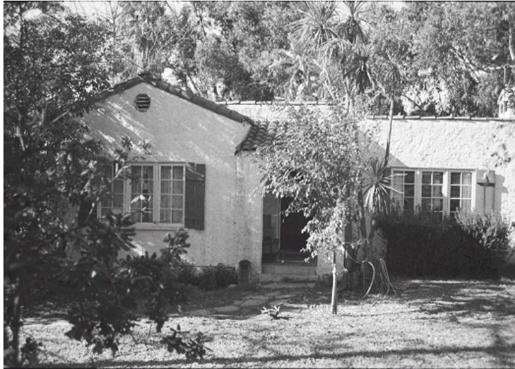
Original survey photo (ca. 1990)
