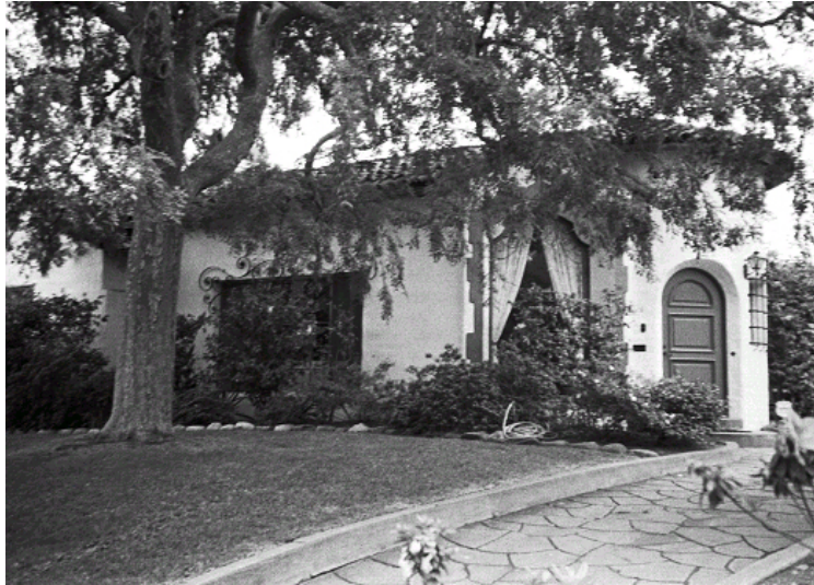
Original survey photo (ca. 1990)
