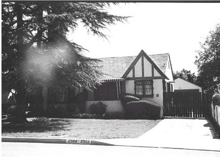
Original survey photo (ca. 1990)
