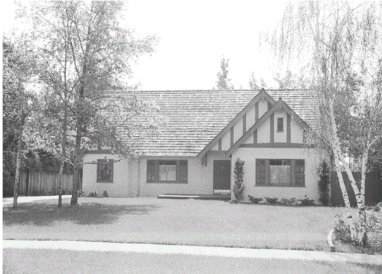
Original survey photo (ca. 1990)
