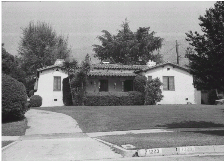
Original survey photo (ca. 1990)
