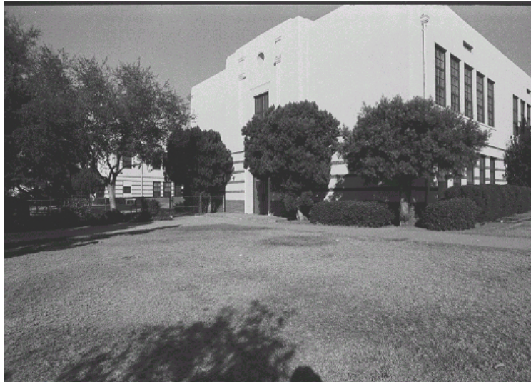
Original survey photo (ca. 1990)
