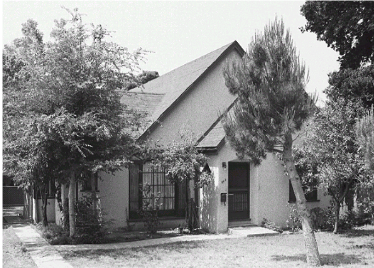
Original survey photo (ca. 1990)
