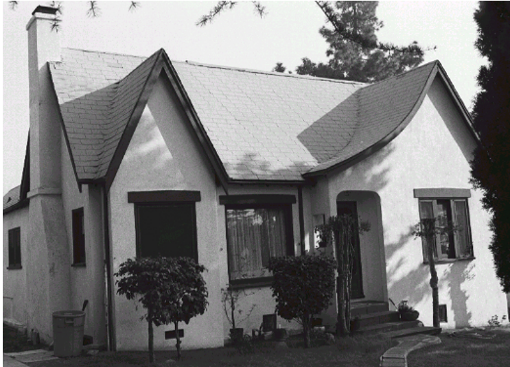
Original survey photo (ca. 1990)
