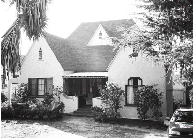
Original survey photo (ca. 1990)
