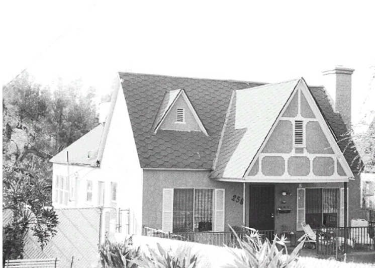
Original survey photo (ca. 1990)
