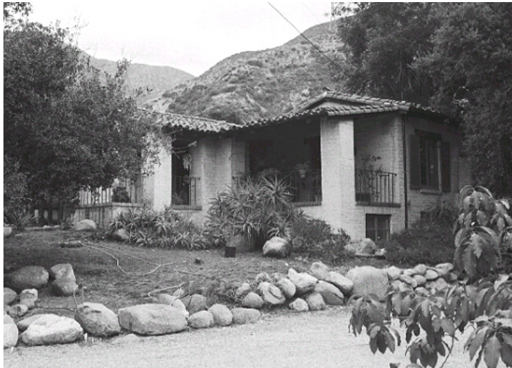
Original survey photo (ca. 1990)
