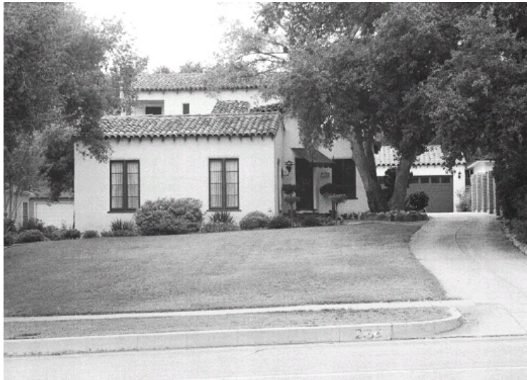
Original survey photo (ca. 1990)
