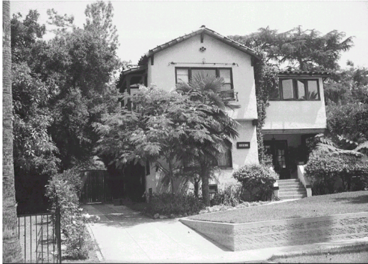
Original survey photo (ca. 1930)
