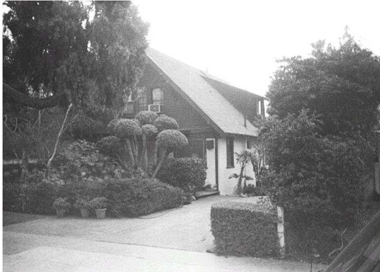
Original survey photo (ca. 1990)
