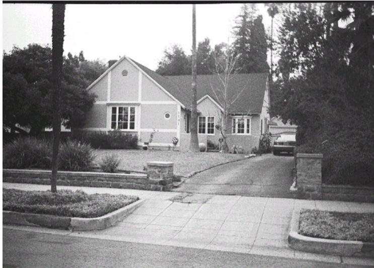
Original survey photo (ca. 1990)
